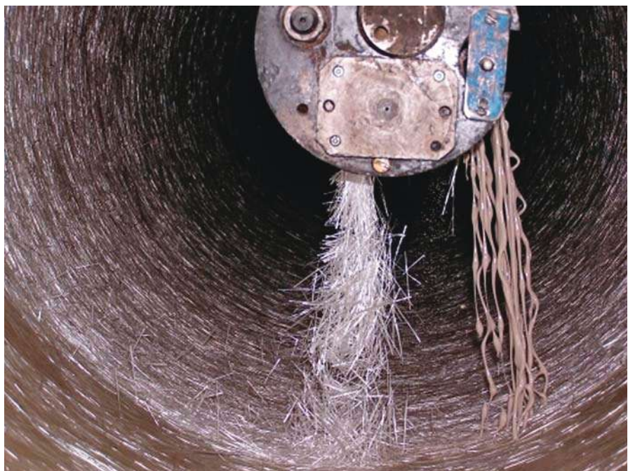
Centrifugal casting of fiberglass-reinforced mortar pipe occurs with materials being placed (glass shown left, resin right) within a rotating steel mold.
