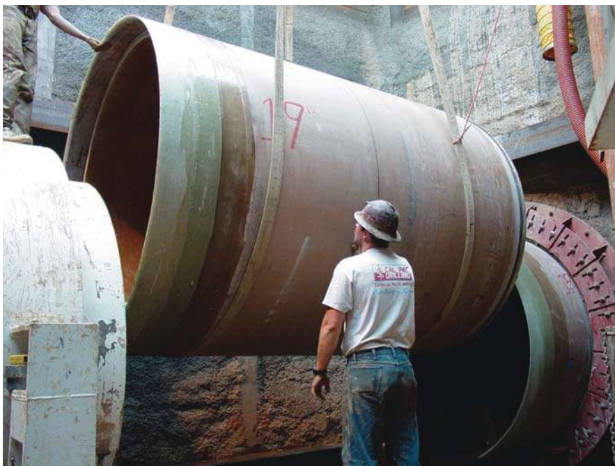
84-in.-diameter 600-ton axial capacity CCFRPM being lowered into the jacking frame.
