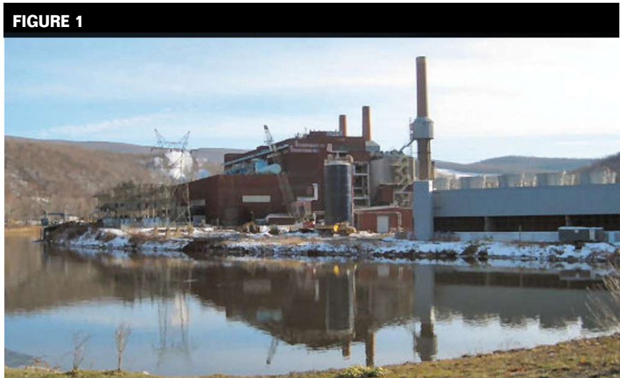
FIGURE 1 The Albright Power Station on the Cheat River in West Virginia.
