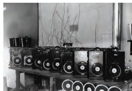
FIGURE 14. A centralized bank of smoked-chart recorders allowed the Electrolysis Department to remotely monitor each bond.
