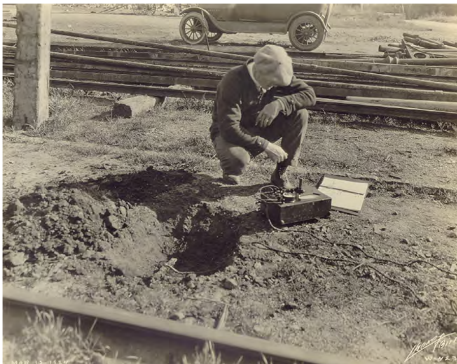
FIGURE 15. An electrolysis surveyor uses a McCollum Earth Current Meter to measure current flow on a buried cast iron pipeline adjacent to a rail line.
