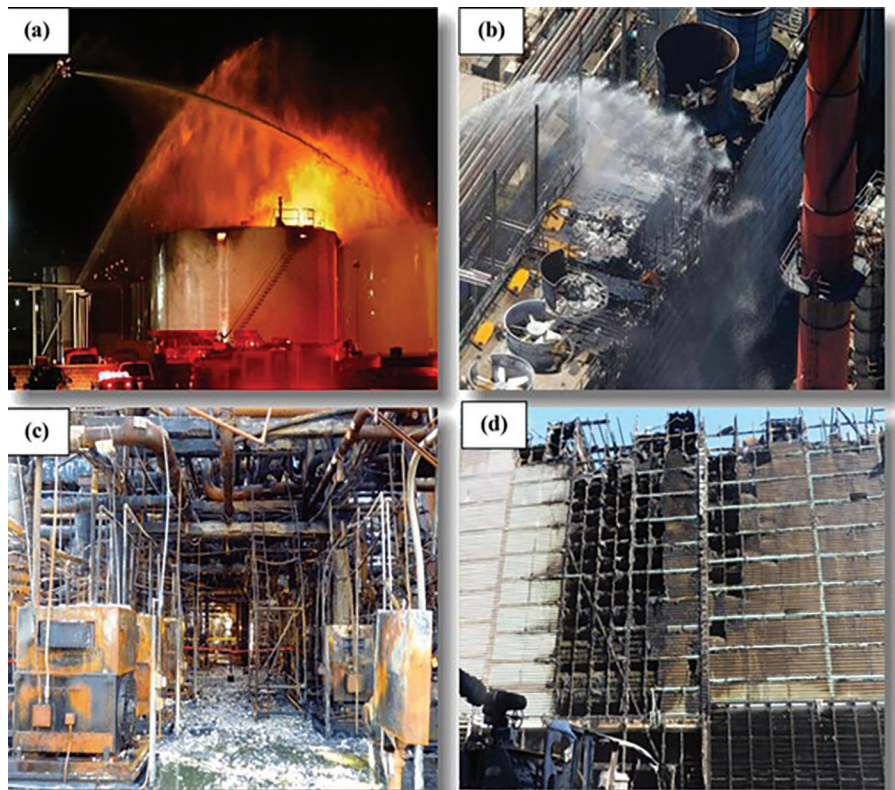
Figure 1 Examples of refinery accidents caused by corrosion failure: (a) Silver Eagle Refinery, (b) Richmond Refinery, (c) and (d) Chevron Refinery.
